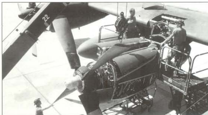
Ground crew prepare to change the Lycoming T56 turboprop engine in the starboard inner position of a Lockheed C-130 Hercules, the complete workhorse of the tactical airlift role in Operations 'Desert Shield' and 'Desert Storm'
