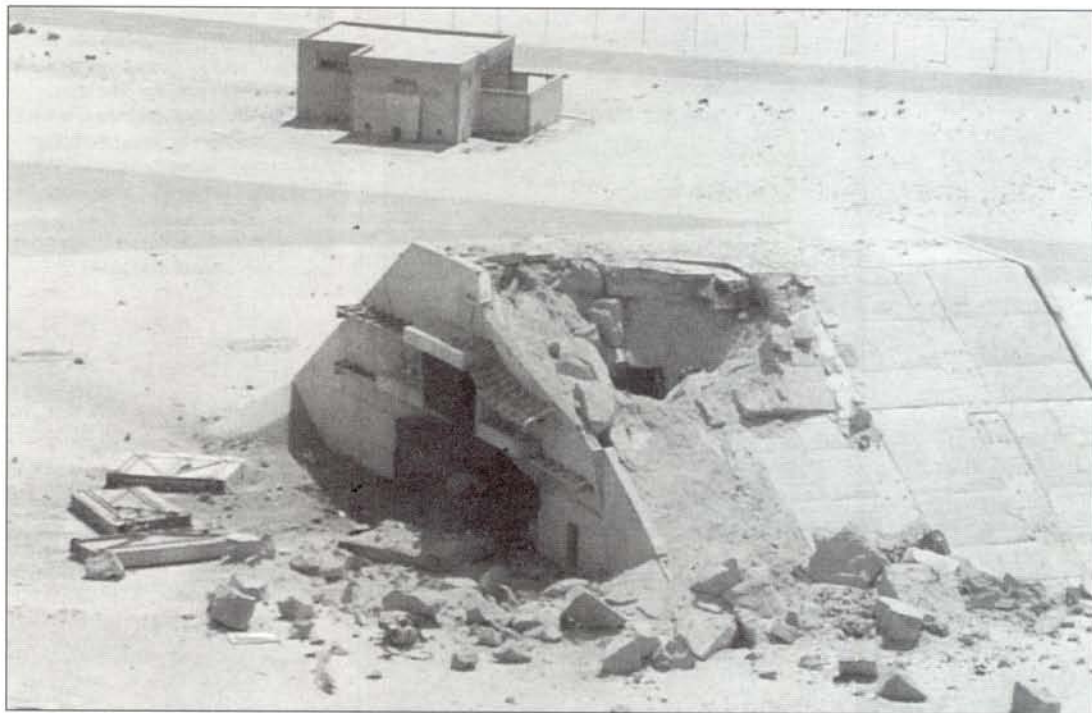
Even Iraq's hardened aircraft shelters, built from reinforced concrete of considerable thickness, proved vulnerable to laser-guided weapons such as the 907 kg (2,000 lb) GBU-10I with its hardened steel casing
